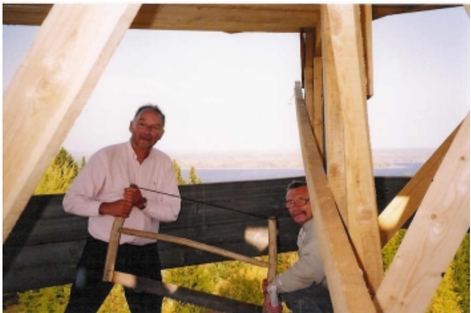
The author (left) helping to repair the 1781 bell tower at Khokhlovka
